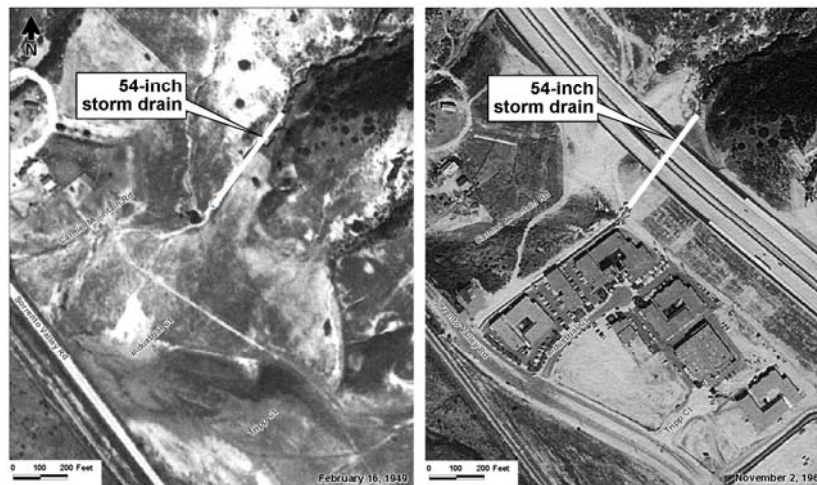
Figure 3. Storm Drain Pre- and Post-Construction of I-5
