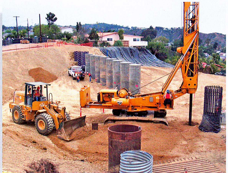
Installation of 54" diameter x 80 ft deep shear pins for Phase 2.
