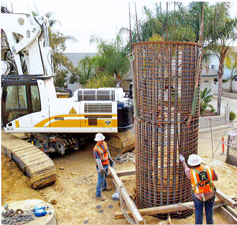
Installation of Phase 3 cages weighing upwards of 42,000 pounds.
