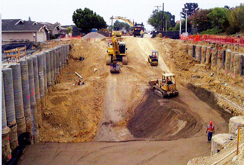
Landslide debris removal and shear pin key construction within the right-of-way.
