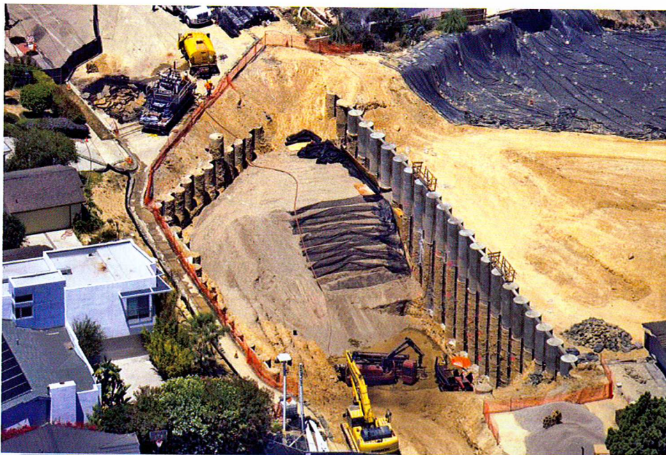
Aerial view of Phase 1 & 2 shear pin construction and slide debris remediation.
